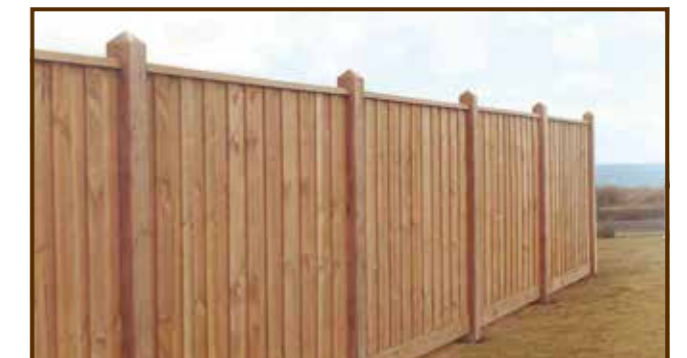
Timber paling fence with exposed posts
